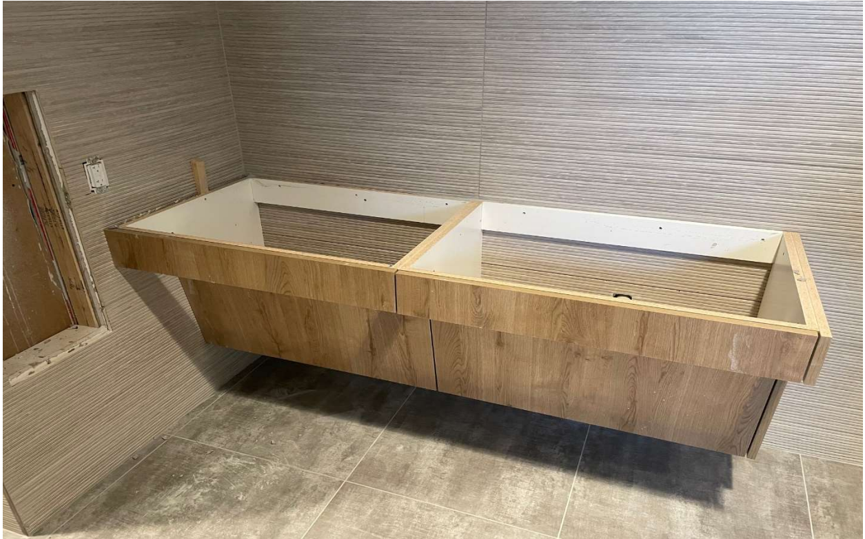
Wall and floor tile in locker room is complete and mill work is being installed.
