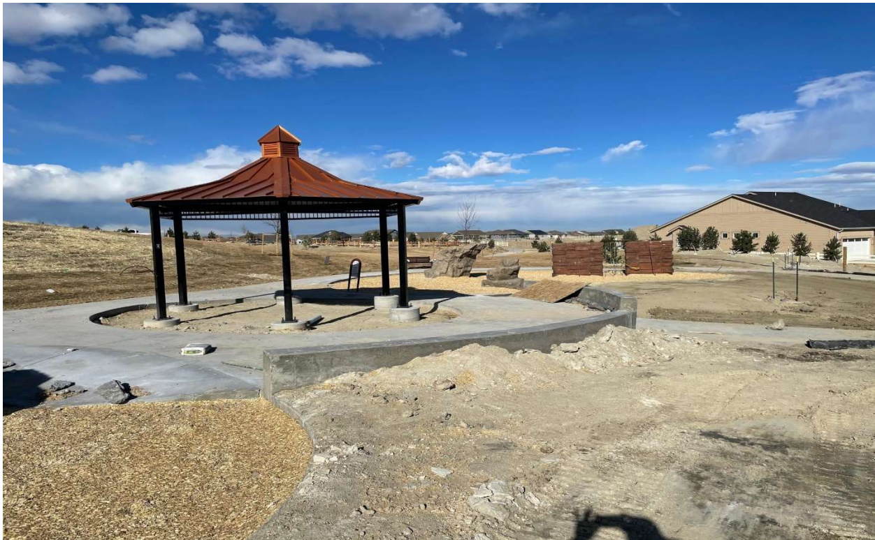
Filing 16 Park with Shade Structure, Benches and Climbing Boulder Installed
