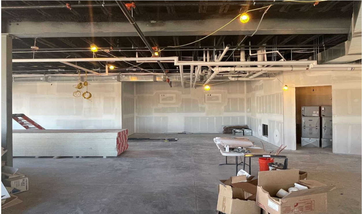
Drywall being installed in lower level of Rec Center
